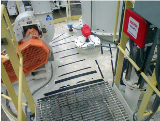
Figure 3. Here, a non-contact sensor sits atop a talc powder vessel to help avoid potential contamination.
