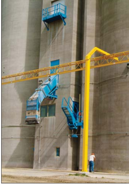
The facility's 60,000-bph bulk weigh loadout scale from C&A Scales is housed inside the slip, in order to protect it and workers from harsh weather much of the year.
