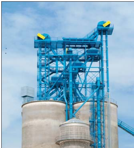
Rooftop structures on top of the slipform concrete elevator include head sections of three Schlagel legs, three Intersystems cleaners, and a Schlagel double distributor.
