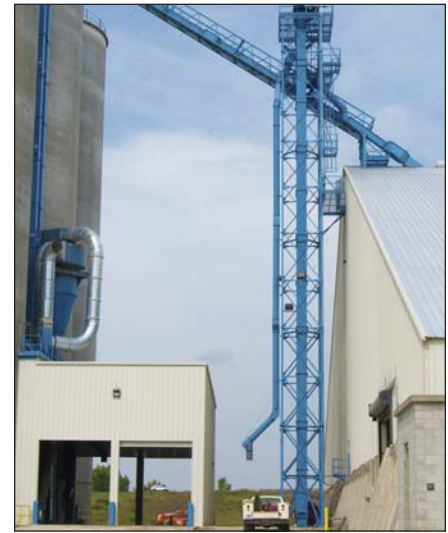
The rebuild also included enclosed truck receiving pits and a dedicated 15,000-bph Schlagel leg and sidewall on the flat storage at right.
