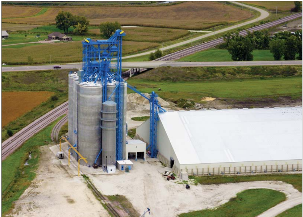
Aerial view of the 1.1-million-bushel replacement grain elevator and adjacent flat storage for Ag Partners LLC along the Union Pacific Railroad at Alton, IA. Aerial photo by JH Photography, Spencer, IA.
