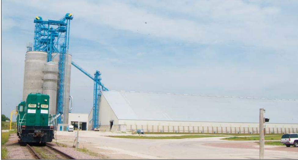
Ground level view of Ag Partners' Alton terminal, which was rebuilt from scratch with the exception of the grain dryer in foreground following a 2008 explosion.
