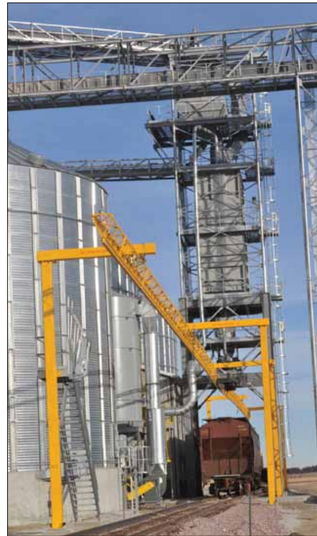
Shuttle trains are loaded by a 60,000-bph Intersystems bulk weigh system topped by a 40,000-bph Intersystems gravity screener all enclosed in an 18-foot-x-18-foot Warrior support tower.
