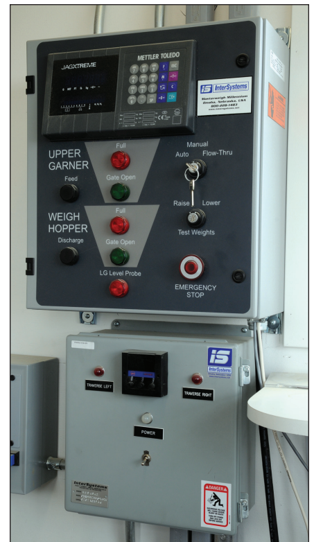
New 50,000-bph Intersystems bulk weigh loadout scale (top) is under the control of an InterSystems Masterweigh Millennium electronic weighing system (bottom).
