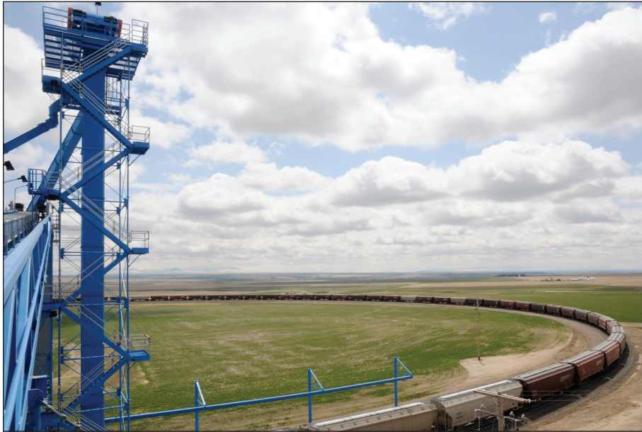
Portion of a loop track allowing an entire 110-car train to be loaded in a single pass without breaking it up for a conventional railyard.
