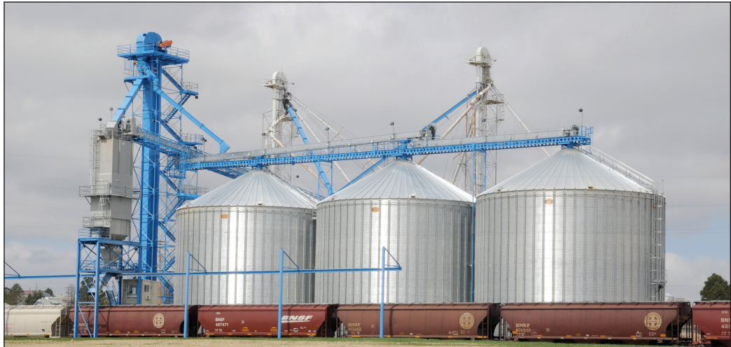
Nearly 400,000-bushel addition with 50,000-bph bulk weigh loadout scale at Columbia Grain International elevator in Carter, MT, to allow facility to load 110-car shuttle trains on the BNSF Railway. Photos by Bruce Selyem.
