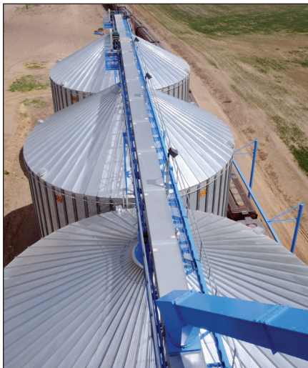
Series of 25,000-bph Intersystems drag conveyors carrying grain out to three new 130,000-bushel GSI corrugated steel tanks.
