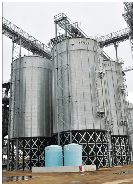
Brock Grain Systems 36-foot hopper tanks at the WFS' new Delavan facility.
