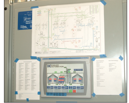
All elevator functions can be controlled from a touch screen inside the master control center.
