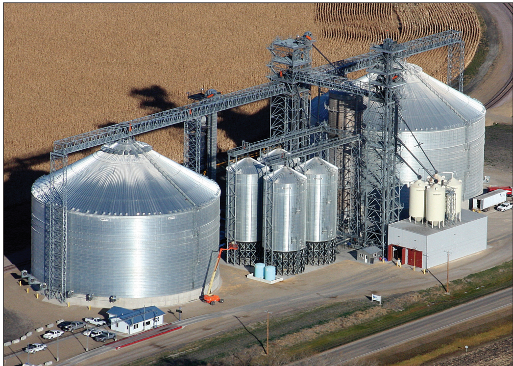
Aerial view of the WFS Delavan, MN, elevator and rail loop track completed just in time for the 2012 harvest which started about a month earlier than normal. Aerial photo by JH Photography, Spencer, IA.
