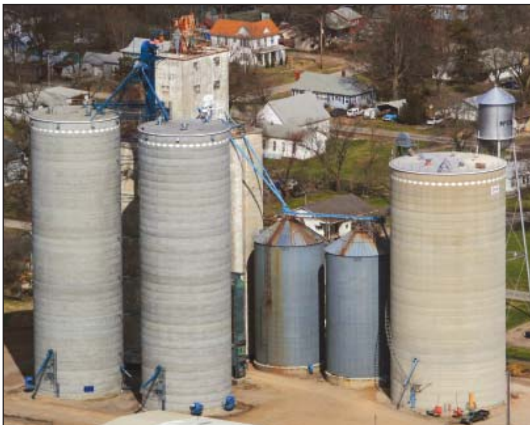
McCune Farmers Union Elevator's single location in McCune, KS. The two new McPherson jumpform concrete at left replace steel storage that was destroyed in a windstorm in May 2009. Photos by Ed Zdrojewski.
