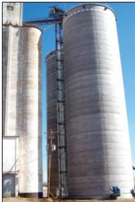
The two new tanks are serviced by Schlagel equipment, including a 15,000-bph leg, 4-hole distributor, and 5,000-bph overhead drag conveyor from the original concrete house.
