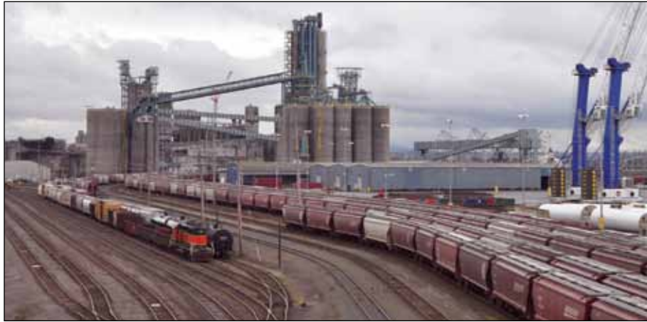
Ground-level view of the terminal from the west, with two new annexes visible in the foreground and a pair of 303-foot Warrior bridges connecting them. Photo by Ed Zdrojewski.
