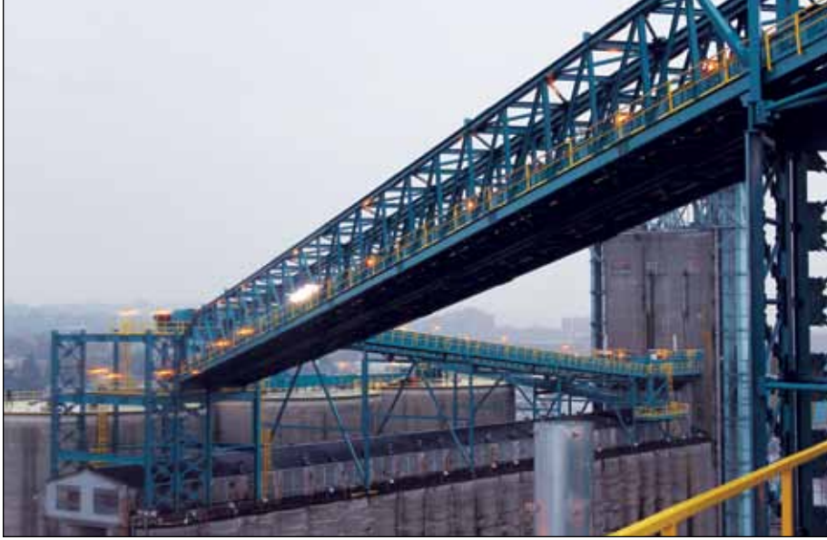
Pair of 303-foot-long bridges are the longest ever manufactured by Warrior Mfg. LLC and carry a set of Hi Roller 54,000-bph enclosed belt conveyors.
