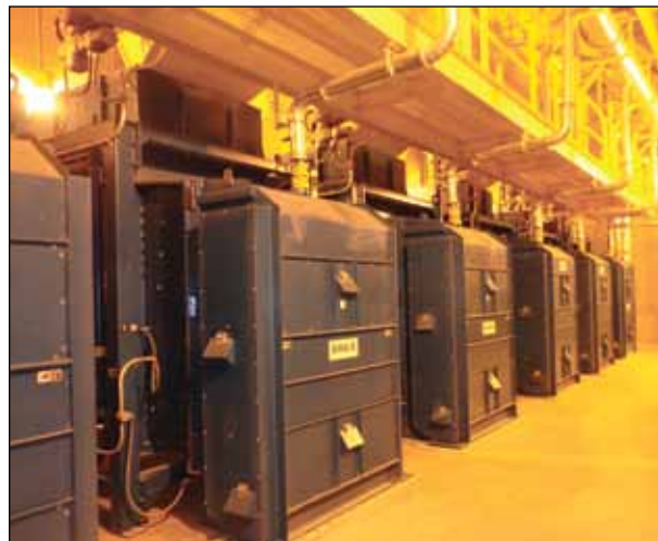
Some of the eight BM&M cleaners in United Grain's new 60,000-bph cleaning house, which has been placed on an annex roof to reduce the number elevations required for grain and minimize damage to the kernels.
