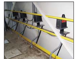
SmartBob-TS1 level sensors measuring Ingredients in micro-bins.
