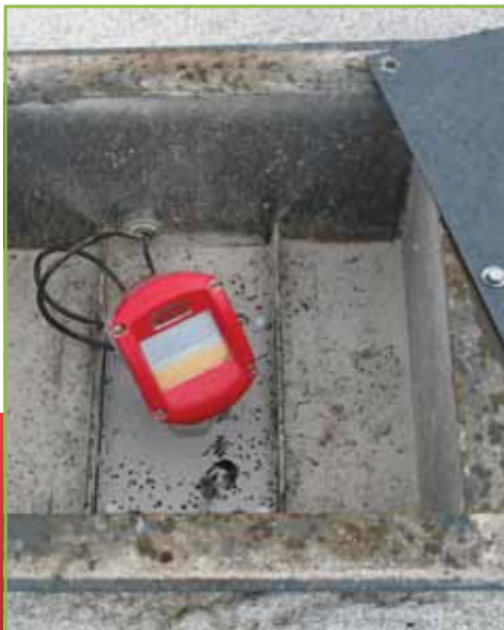
Scanner was mounted into an existing opening.
