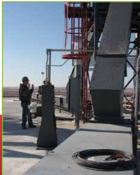
Top of silo with gravity on conveyor fill.
