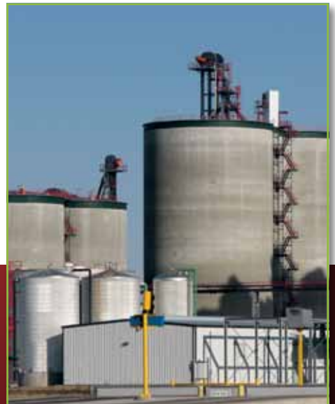
3DLevelScanner is now installed on all four large silos.
