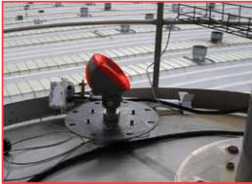
Dust penetrating, non-contact device is easy to install.
