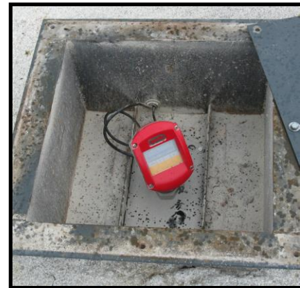
Scanners are installed on all 4 large silos.
