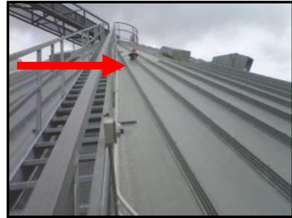
Scanner #1 mounted near the center of the bin, but away from the fill stream.
