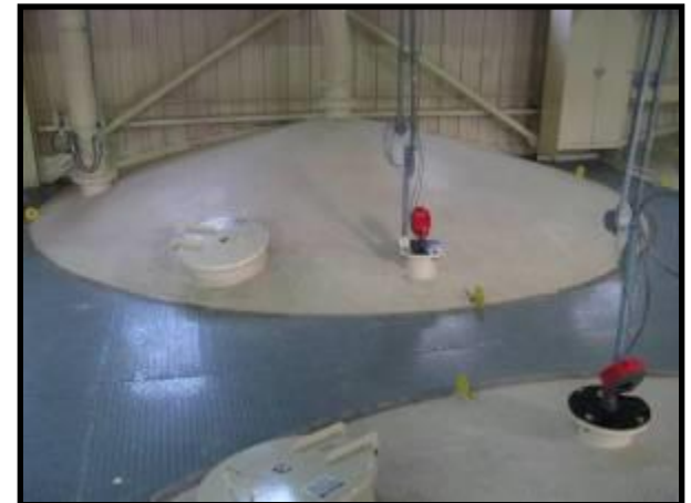
Scanners are installed on 21 silos.
