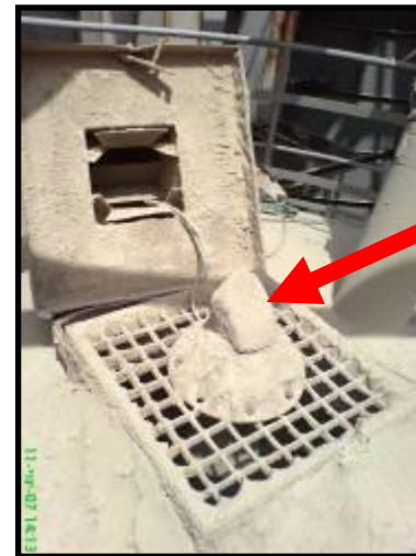
Flour mill install
