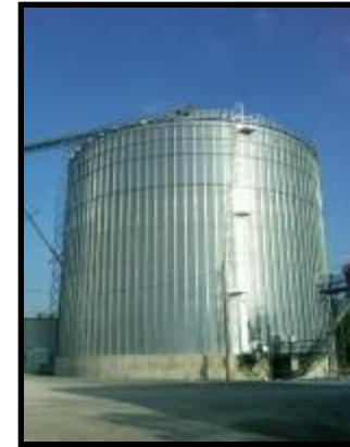
Grain Bin Installation
