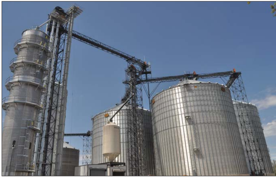
The Delhi facility, from left: 4,800-bph Zimmerman tower dryer; two Schlagel legs, a 15,000-bph receiving leg and a 10,000-bph dry leg; 12-foot-x-12-foot-x-150-foot Warrior tower; 75,000-bushel Sukup wet tank visible behind the tower; two receiving pits, one of them new; grain storage complex, with one of two new 515,000-bushel Sukup tanks visible at far right.
