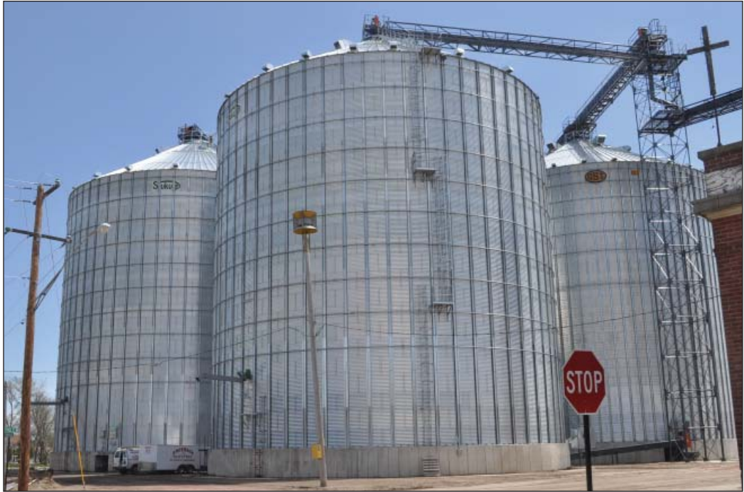
Two new 515,000-bushel Sukup corrugated steel storage tanks effectively double storage capacity at Meadowland Farmers Cooperative's branch elevator in Delhi, MN. Photos by Ed Zdrojewski.
