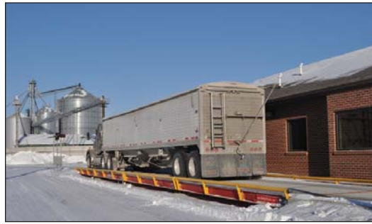
An incoming grain truck is weighed on an 80-foot Fairbanks scale, one of two adjacent to the new office building constructed during the upgrade.
