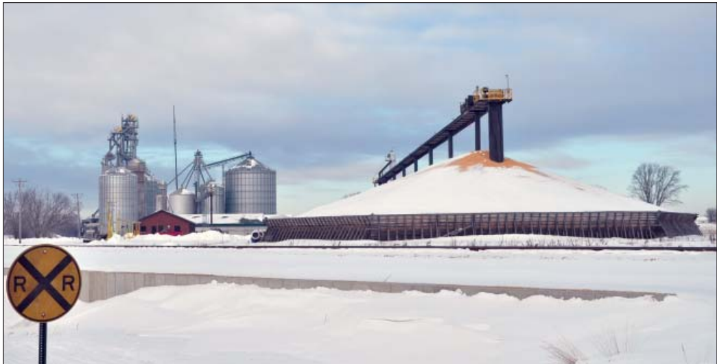
A new 2-million-bushel temporary storage pile in the foreground is part of a major upgrade completed in October 2013 at Gavilon Grain's recently-acquired elevator at Avalon, WI, which also includes 1.2 million bushels of upright storage. Photos by Ed Zdrojewski.
