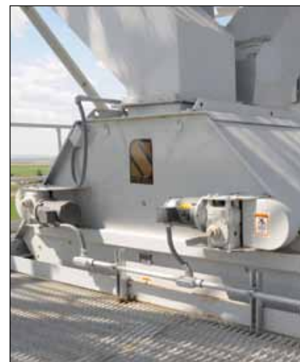
Seven-duct Schlagel SwingSet distributor can send grain to storage, dryer, or truck loadout.
