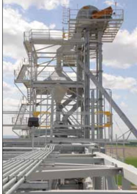
Equipment atop the LeMar support tower includes a J & D 20,000-bph gravity screener and Schlagel double distributor.
