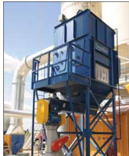
Dust emissions are kept under control with a Donaldson Torit baghouse system.
