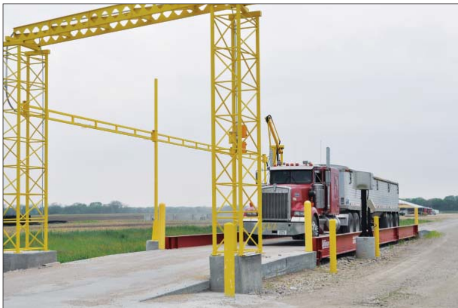
Truckers pull onto a Rice Lake outbound scale, which is outfitted with Comco scale automation and a Gamet truck probe.
