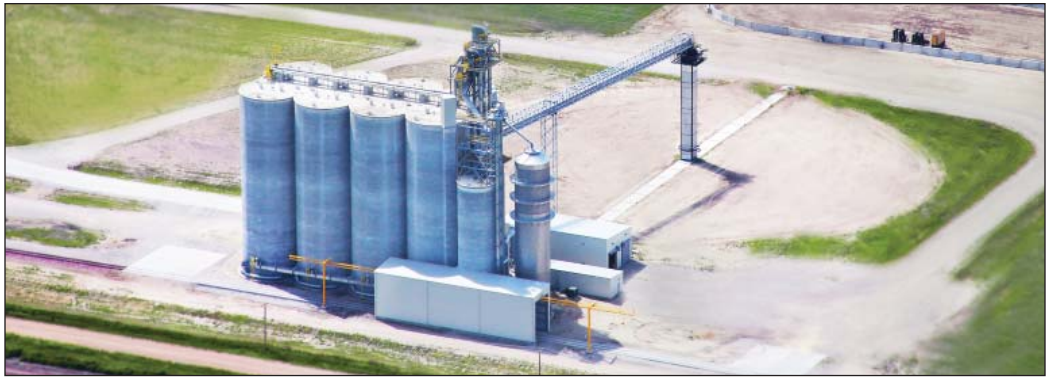
The new Superior East, LLC rail terminal near Superior, NE includes a 1.25-million-bushel slipform concrete elevator in foreground and a 2.2-million-bushel center-fill ground pile behind. Not visible are two 975,000-bushel oval ground piles. Aerial photo by Ink Photography.
