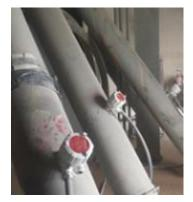
One large facility recently installed the Flow Detect 2000 on the legs of its distributor. When the sensors were first put into operation, one sensor alerted that material was still flowing through a leg after the gate was shut.
