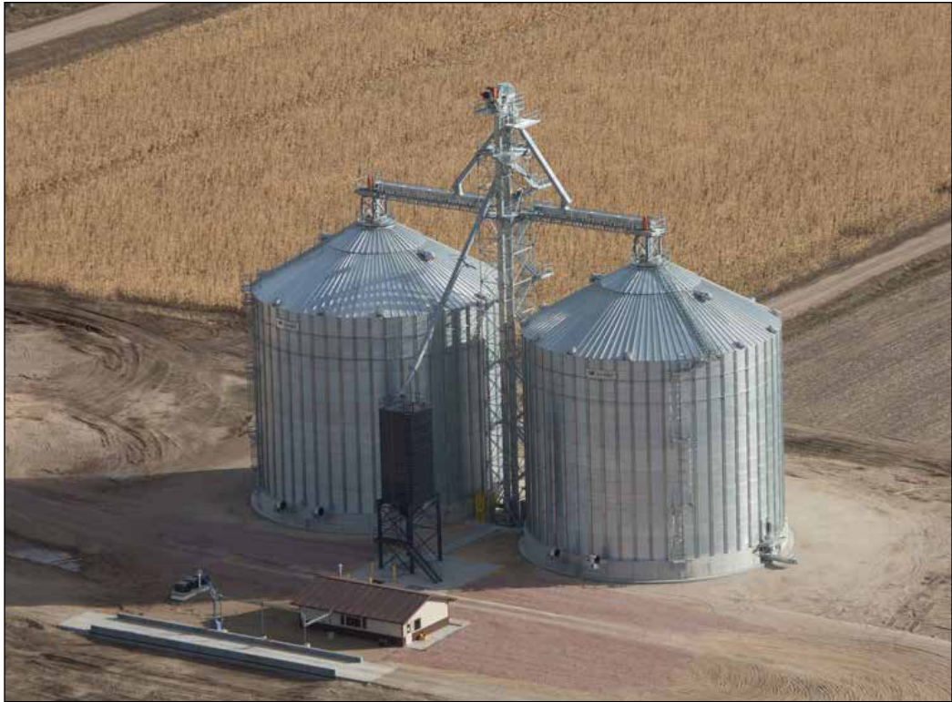
Farmers Cooperative Elevator Co.'s new Mirage Flats 620,000-bushel all-steel elevator near Hay Springs, NE handles grain from a surrounding irrigation district. Aerial photos courtesy of EBM Construction Inc.
