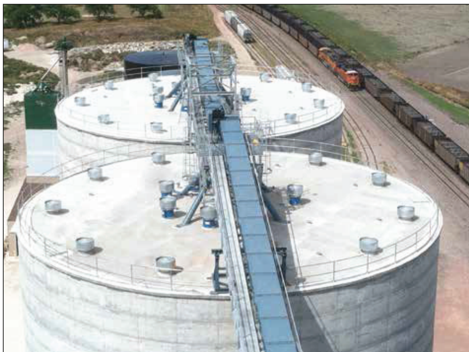
New overhead Hi Roller 20,000-bph enclosed belt conveyors carry grain out to the two newest jumpform concrete tanks at Hemingford.
