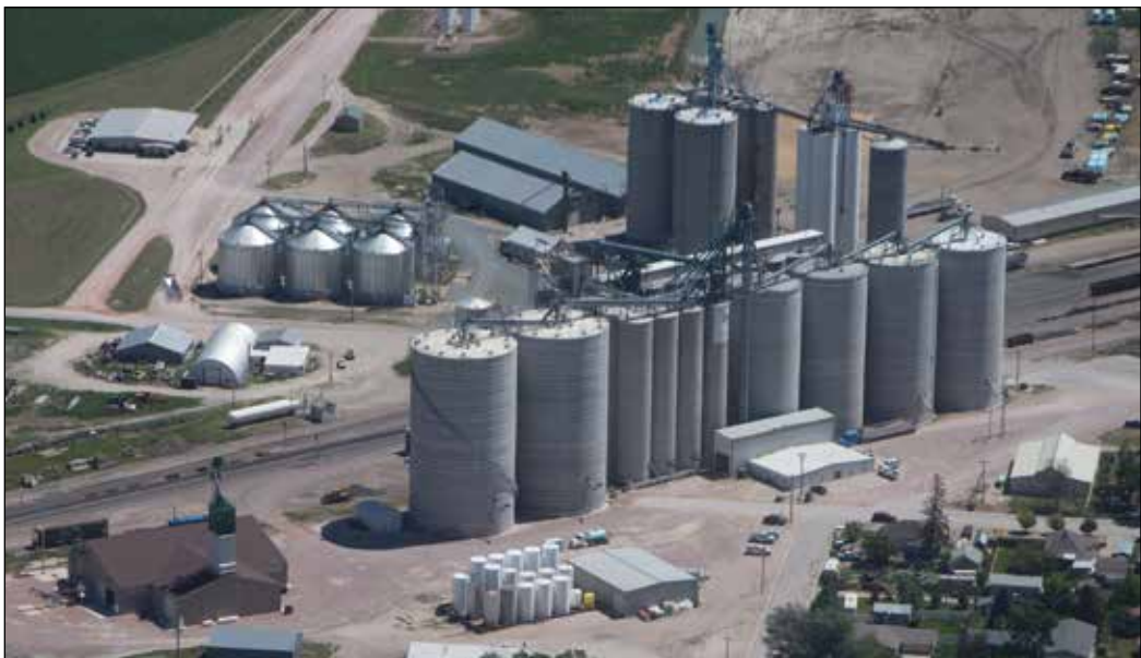
The cooperative's flagship elevator in Hemingford, NE with two new 500,000-bushel jumpform concrete silos near the center of the photo.
