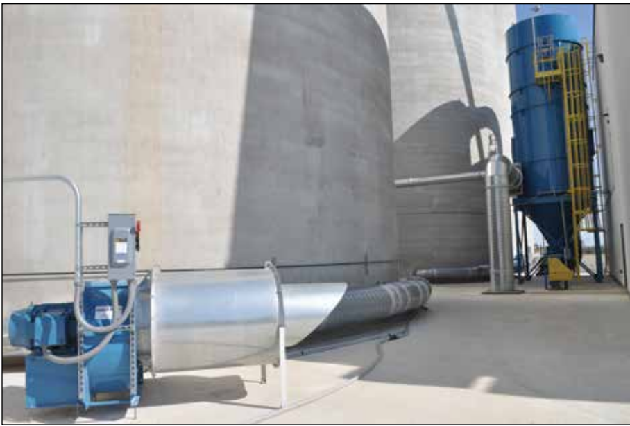
AIRLANCO Airauger aeration and unloading system at left is powered by 75-hp centrifugal fans. AIRLANCO baghouse filter at right services the facility's two truck receiving pits.
