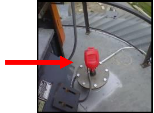
Scanner #1 mounted near the center of the bin.
