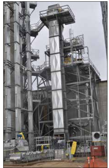
InterSystems 60,000-bph shipping leg deposits grain onto an overhead 60,000-bph covered belt conveyor out to the river.
