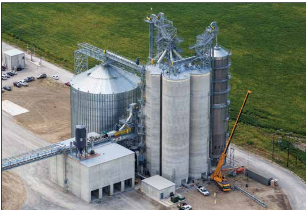
Louis Dreyfus Company's new 800,000-bushel river terminal at West Memphis, AR sends grain more than half a mile via covered belt conveyor (left) out to moored barges. Photo by Aerial Innovations of Tennessee, Nashville.
