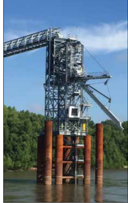
Warrior stair tower over the water supports a Warrior/Micada surge bin and a Premier Fabrication loadout spout. A covered belt conveyor running more than half a mile in a Warrior box bridge brings grain from the elevator. Photo from Louis Dreyfus Company.
