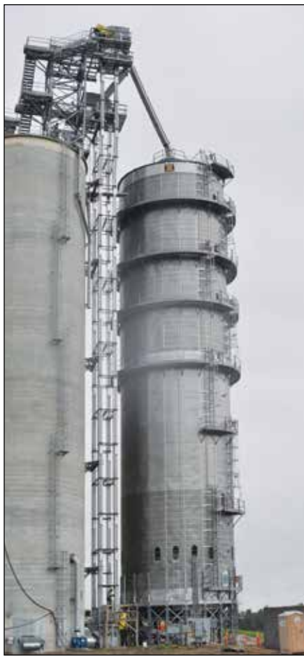
New 12,000-bph Zimmerman continuous-flow tower dryer, the largest that manufacturer makes, is serviced by 15,000-bph InterSystems wet and dry legs.
