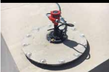
Radar can be mounted on flat or angled roofs and in segmented silos
