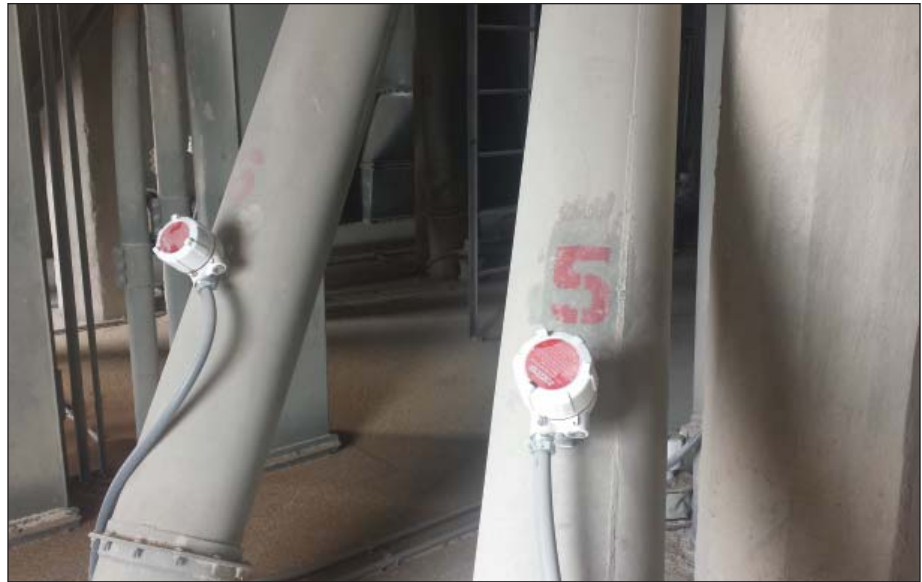
Photo shows a feed mill distributor where product cross-contamination potentially could occur. The placement of a BinMaster Flow Detect 2000 single-piece flow detector ensures product flow has stopped completely. Photos courtesy of BinMaster.
