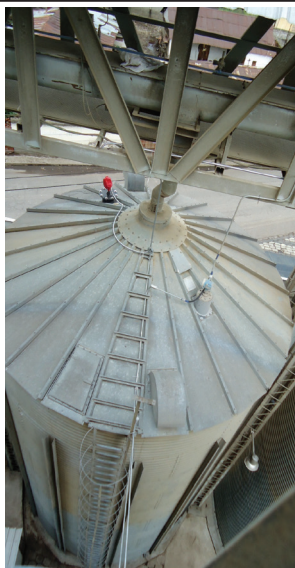
Silos can be challenging structures to measure and often they come with some surprises that need a work around.
