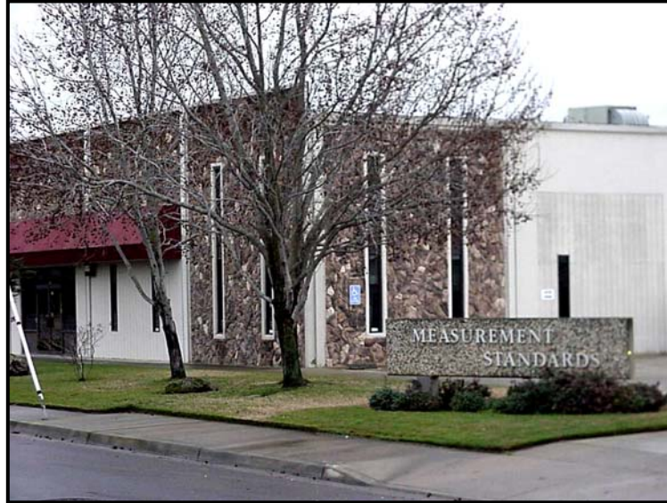
Division of Measurement Standards Building 8500 Fruitridge Road, Sacramento
