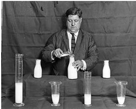
Testing Milk Bottles for Legal Capacity
